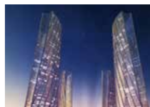
Lusail Tower, Qatar - HDPE
