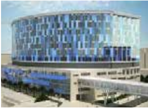
Al Amiri Hospital, Kuwait - Sanit & HDPE
