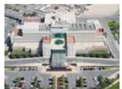
Saudi German Hospital Dammam, KSA - Wefatherm
