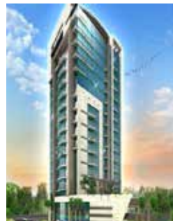
Al Noor Tower Abu Dhabi, UAE - Wefatherm & Sanit
