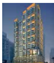
Wafra Tower, Reem Island, UAE - Marley & HDPE
