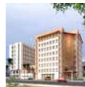
National Hospital, Riyadh, KSA - Wefatherm
