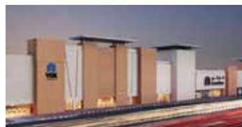
Sharjah City Center Expansion & Refurbishment, UAE - Marley
