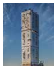
La Plage Tower, UAE - HDPE
