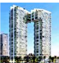
Kifaf Tower, UAE - Wefatherm & Sanit
