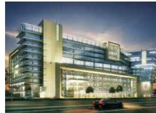
AMAF Headquarter building, Dubai - Wefatherm
