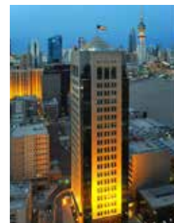
Shaab Tower, Kuwait - HDPE
