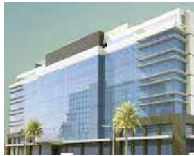
Anfas Al Raha Hospital KSA - Wefatherm Sanit
