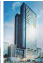
Crowne Plaza Dubai Marina, UAE - Sanit
