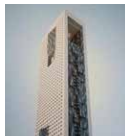
Gate Tower Al Khan, UAE - Marley
