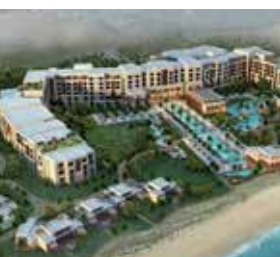
Park Hayat Sadiyaat, UAE - HDPE
