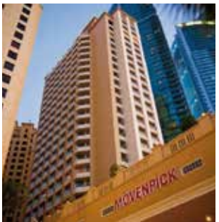
Movenpick Hotel JBR, UAE - Sanit
