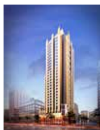
Park Inn Hotel in JVT, UAE - Marley
