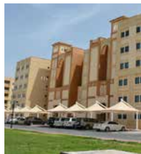
Ruweis Housing Complex, UAE - Sanit
