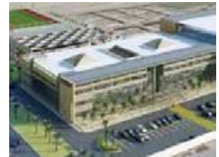
American International School Jeddah, KSA - Wefatherm
