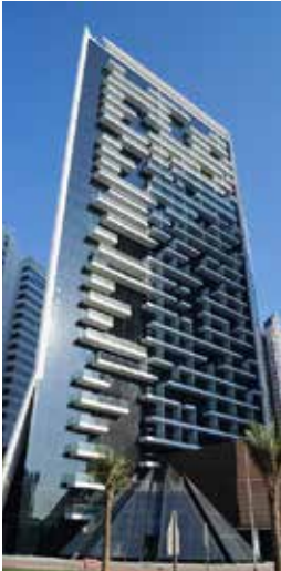
Marquise Tower, UAE - Wefatherm
