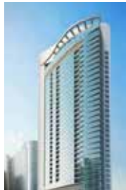
Corniche Tower, UAE - Wefatherm
