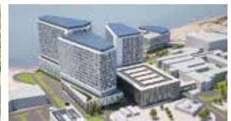
New Maternity Hospital Kuwait - HDPE
