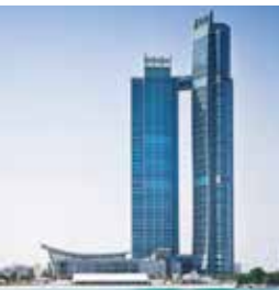
Nation Towers, UAE - Studor
