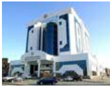
Dar Alshifa Hospital, Kuwait - HDPE
