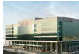
Dr. Suleiman Habib Hospital, KSA - Wefatherm
