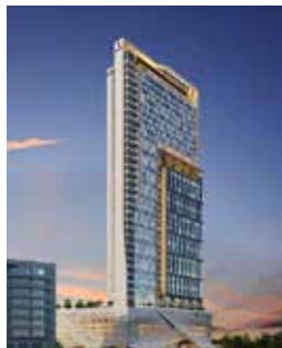
Hilton Double Tree Jeddah, KSA - Sanit
