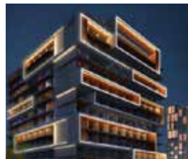
Aloft Hotel, Palm Island, UAE - Sanit
