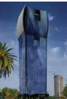
Al Khaleej Towers, Qatar - Wefatherm
